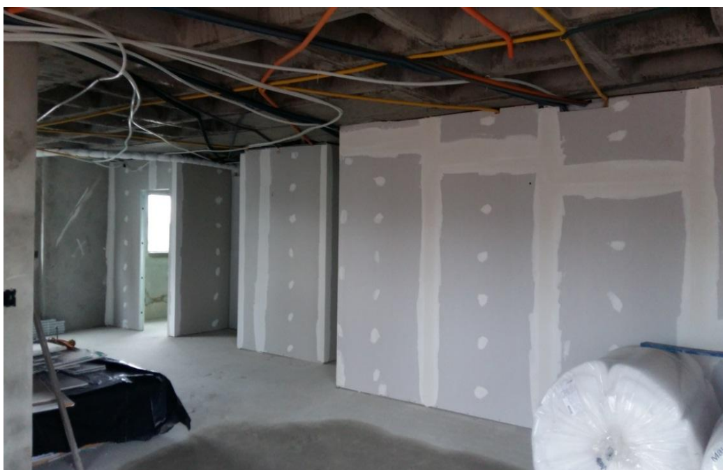
Fig. 7: Arrangement of the plaster in the apartment
