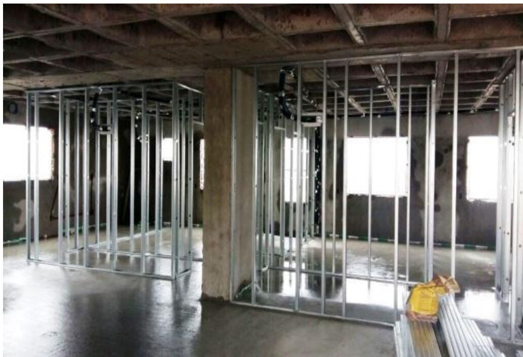
Fig. 6: Arrangement of the plaster in the apartment
